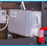
A Pumped Main Drainage System Pumps The Waste Water From The Drip Tray Over A Distance Of 100m & A Rise Of 5m. (Factory Installed)
