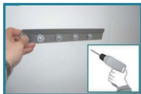
Fix Wall Mounted Bracket to Wall
